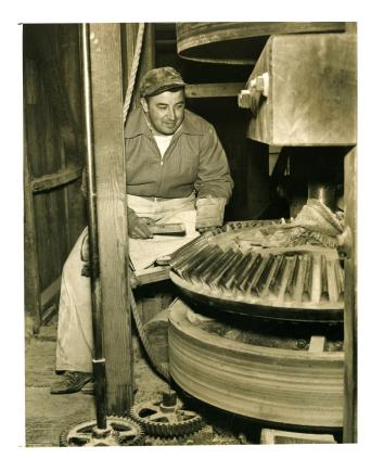
Addison Krom is shown repairing wooden cogs on a turbine shaft in 1953.
