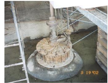
*Mill water turbine exposed during initial restoration.*
